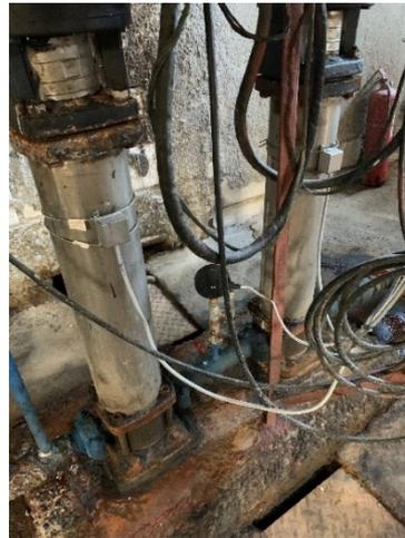
Fig. 1. One pair of pumps with sensors attached.
